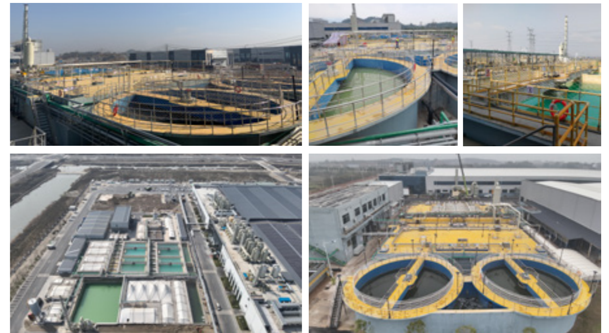
Wastewater Treatment Facilities
