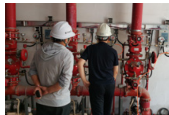
Special Hazard Inspection
